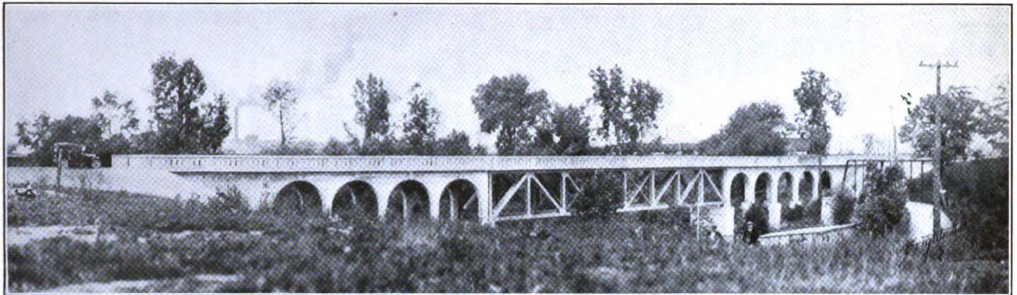
Photo From Michigan State Highway Department 1918 Biennial Report Showing The Newly Completed Bridge Digitized By Google and Enhanced By HistoricBridges.org
